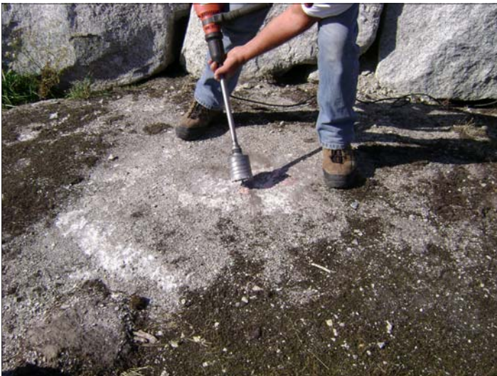
District of Sechelt Public Works Department installs monuments.
